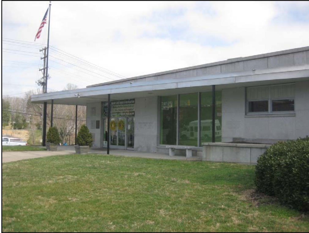
Photo 3: Façade of Reeves Community Center, West Elevation
