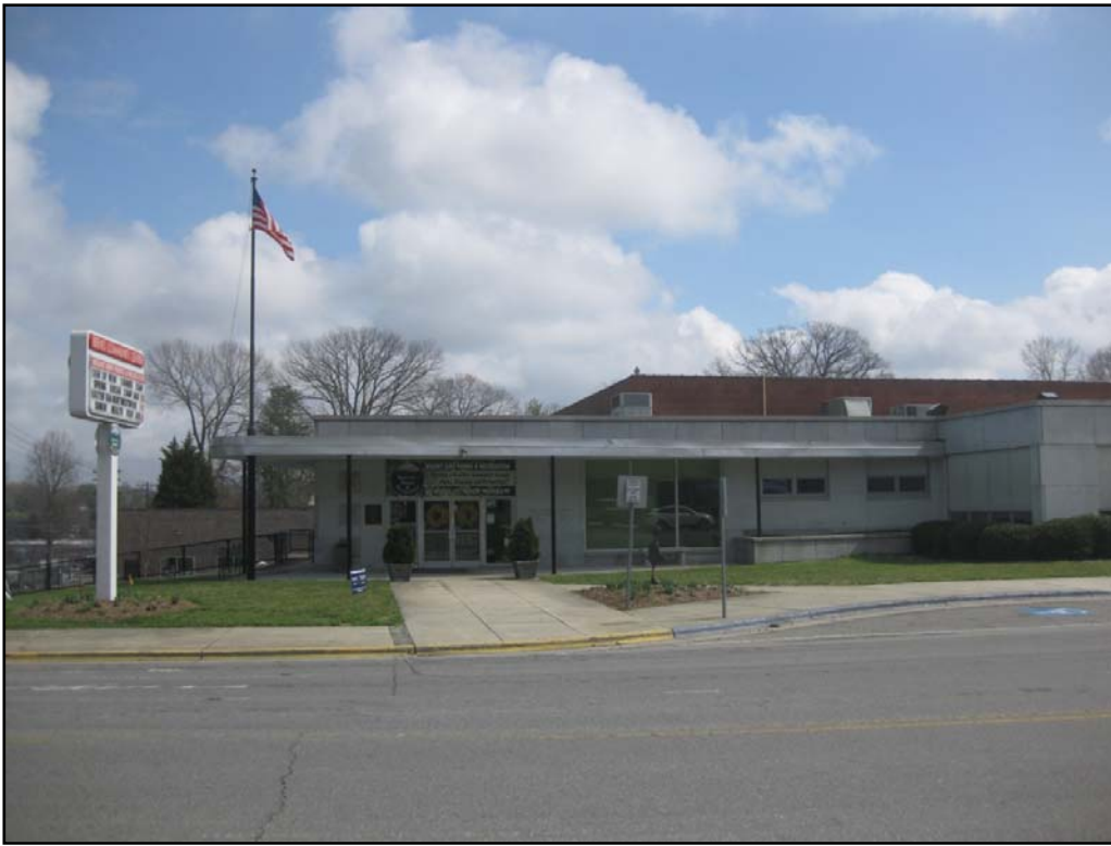
Photo 1: Facade of Reeves Community Center, West Elevation
