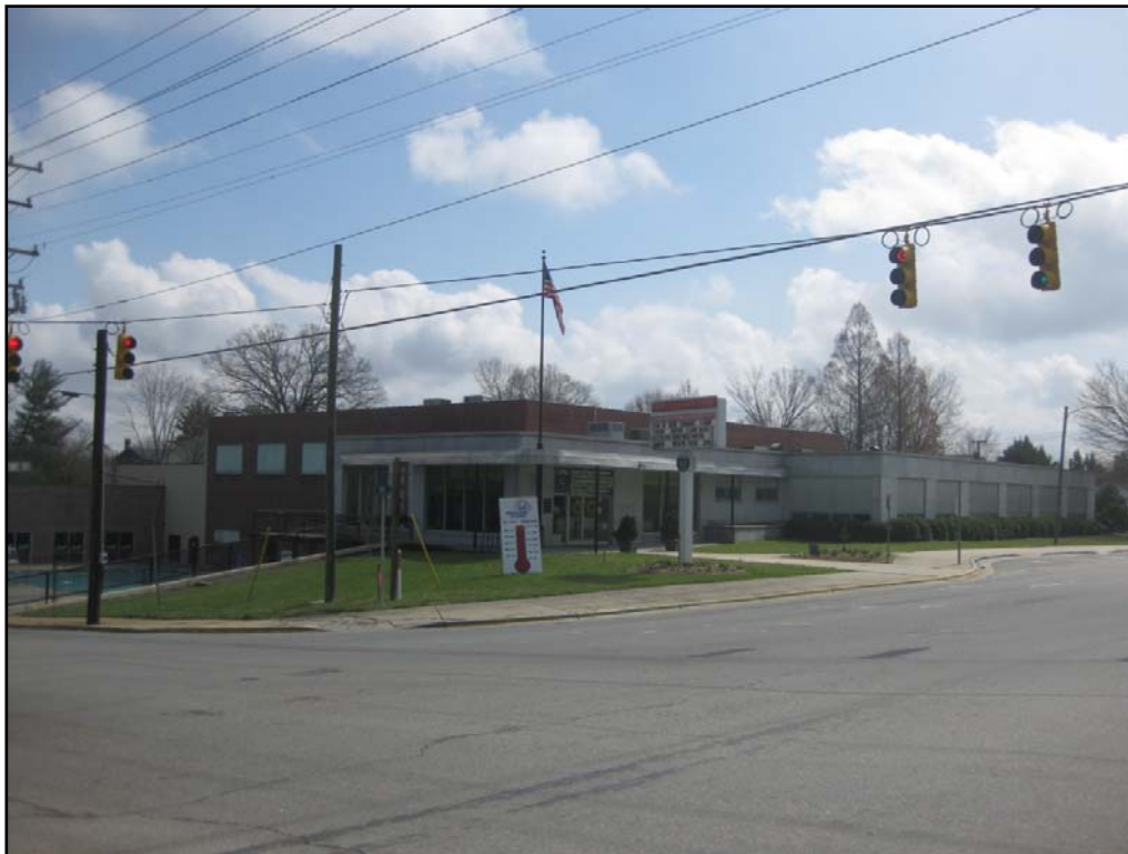
Photo 2: Façade of Reeves Community Center, oblique view of North and West Elevations
