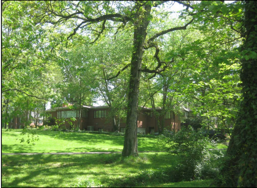
Photo 27: House, 227 Grace Street
