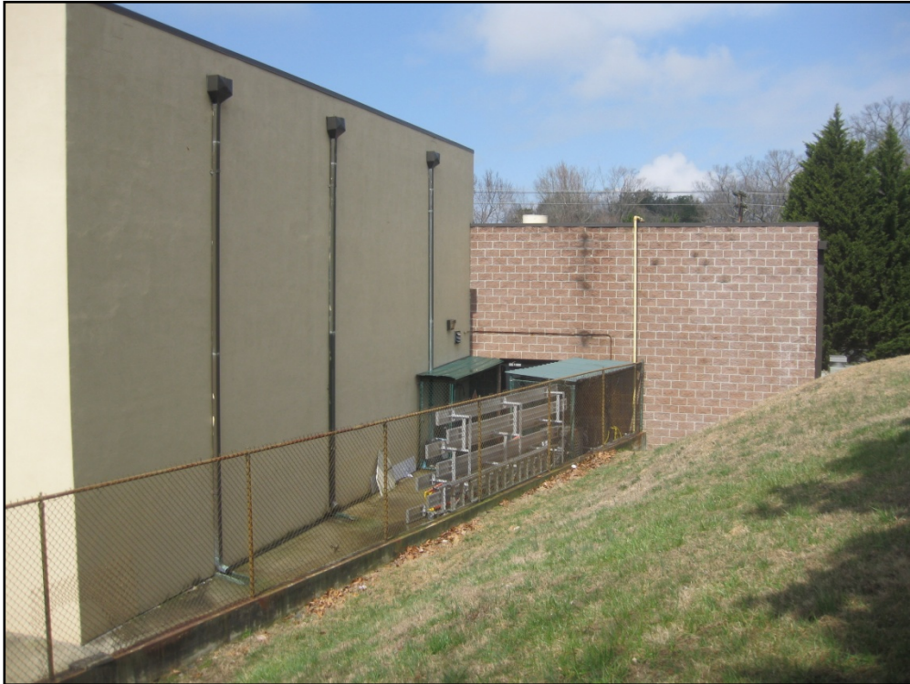
Photo 6: Reeves Community Center, Hyphen, East Elevation
