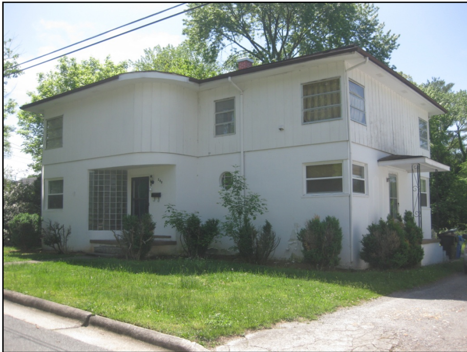
Photo 28: Franklin Boyd House, SR0270 209 West Oakdale Street
