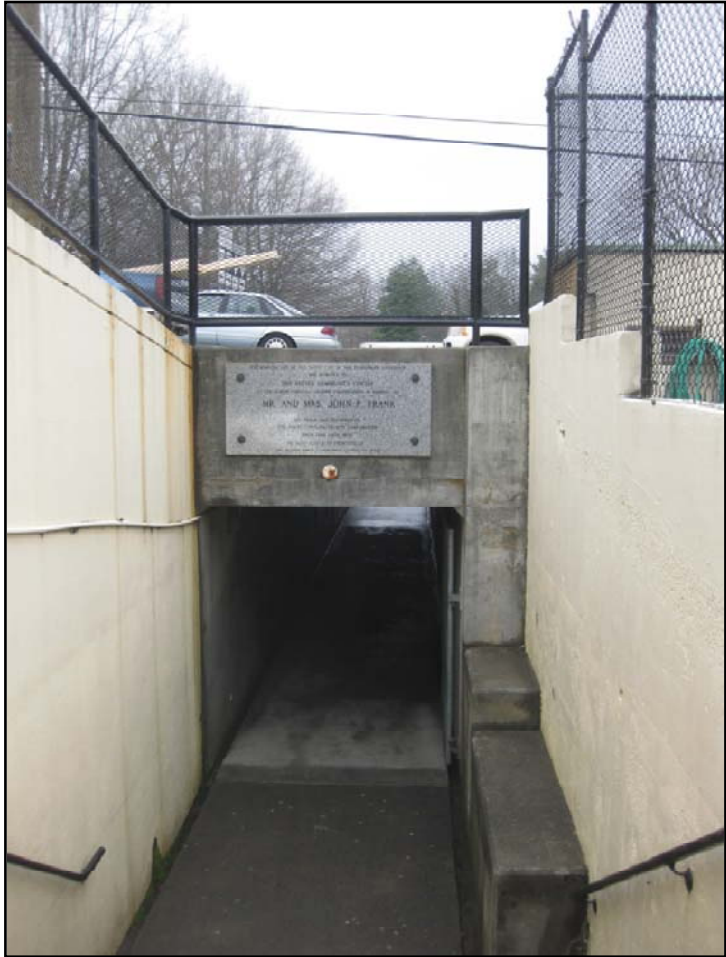
Photo 10: Reeves Community Center, Underpass
