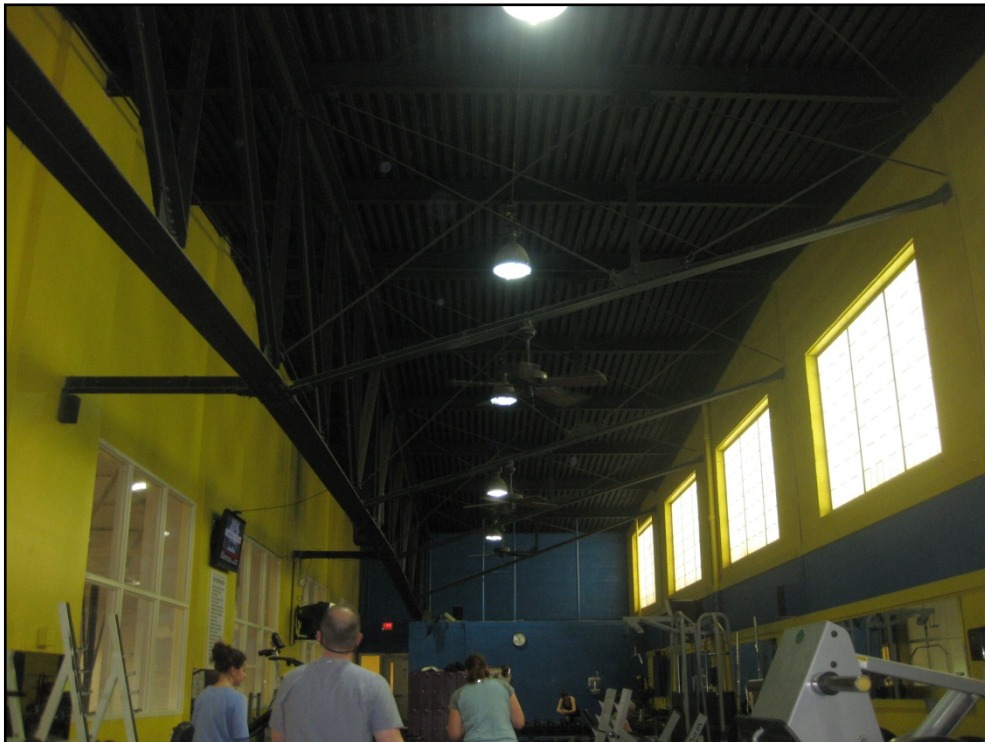
Photo 14: Reeves Community Center, Enclosed Balcony/Fitness Room
