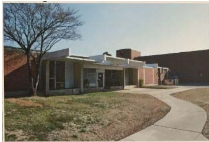
Photo 25: South Main Street YMCA (GF2991) 401 South Main Street, High Point 2009, HPO Survey files
