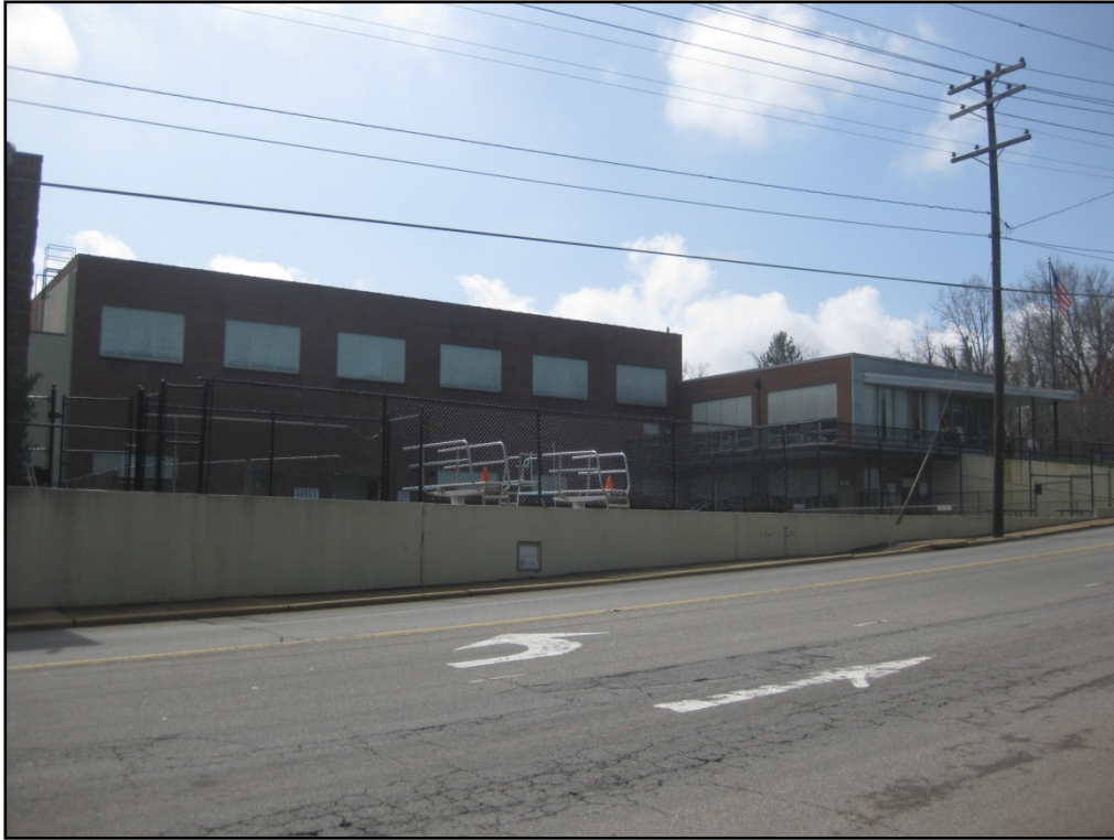
Photo 8: Reeves Community Center, Pool Enclosure and Gymnasium, North Elevation
