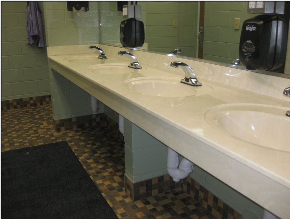
Photo 16: Reeves Community Center, Locker Room, typical fixtures and finishes
