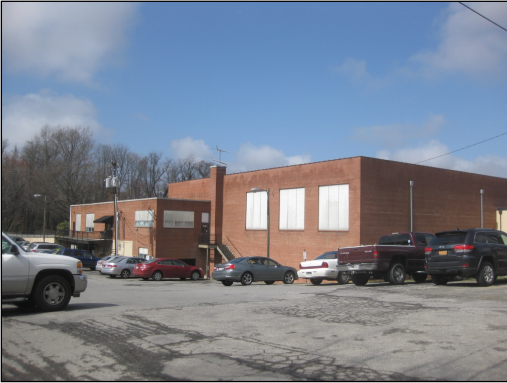
Photo 4: Reeves Community Center, South Elevation
