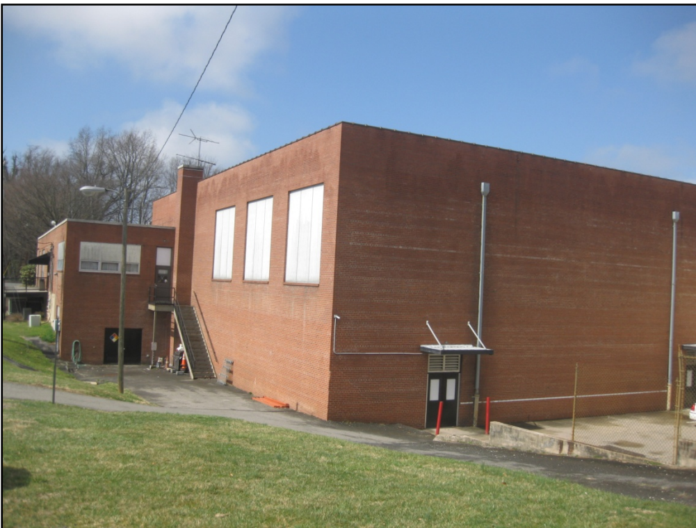
Photo 5: Reeves Community Center, Oblique Rear of Gymnasium
