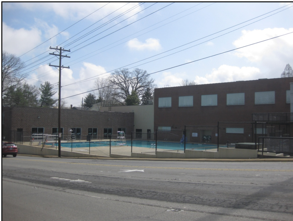
Photo 9: Reeves Community Center, Outdoor Pool and Gymnasium, North Elevation
