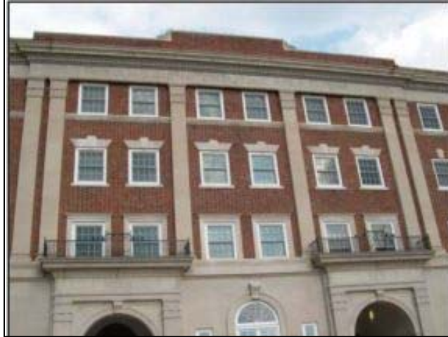
Photo 20: Former Spruce Street YMCA (FY0800) 315 North Spruce Street, Winston-Salem Photo courtesy Forsyth County Historic Resources Commission Files
